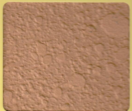
SEMI GLOSS EMULSION AS TOP COAT E 1426 BY HOPPER GUN HEADCUT
